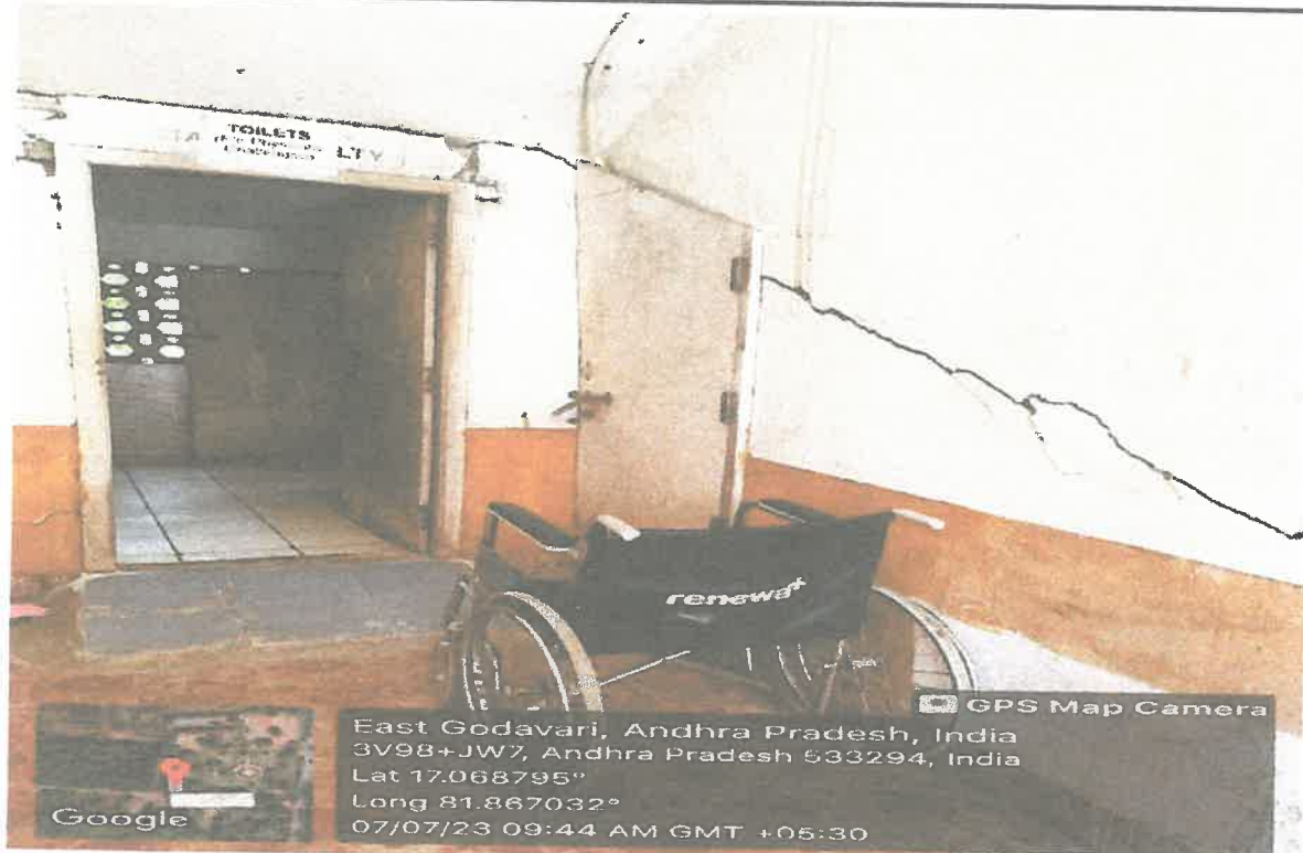
Physically Challenged Toilets
